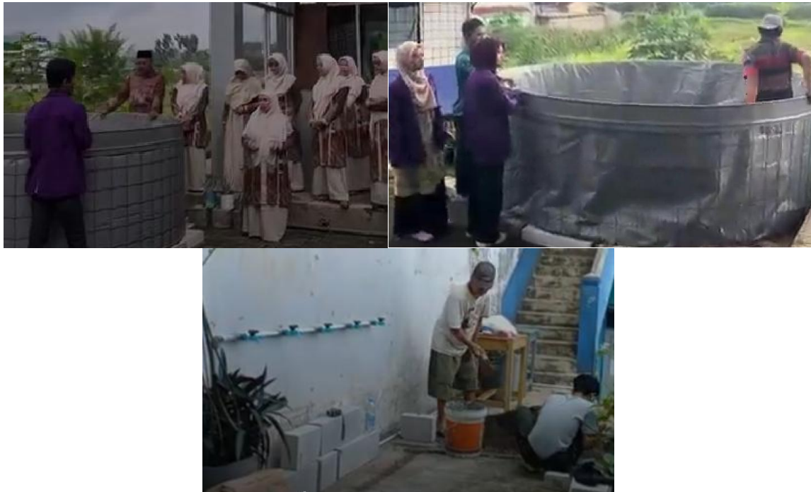
Figure 1. Ablution Water Installation and Fish Pond
